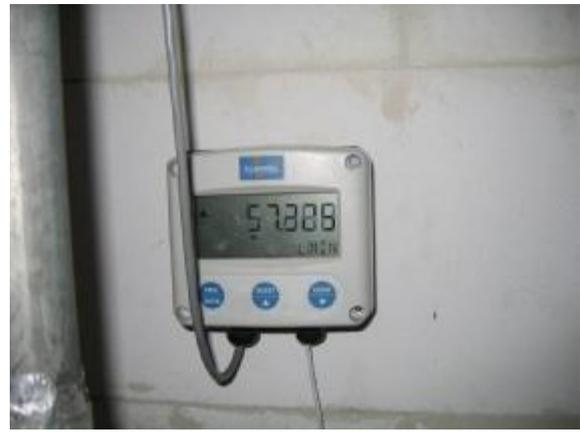
Sprinkler flow-rate meter
